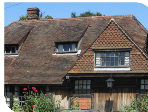
Clay tile roofs and tile-hanging
